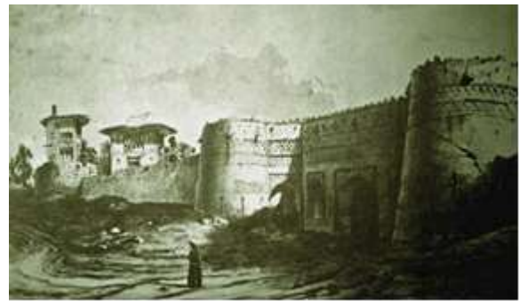
Figure 6 & 7. Physical structure of Boroujerd (19 th century, top) and wall and towers of Boroujerd in Islamic period (Century 10 AH, bottom) (Authors).
